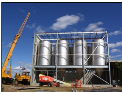
400-Barrel fermentation vessels.
